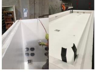
IMRAE CoatMasters® Elastomeric Coating can be easily applied, by either roller or spray, for quick set-up and clean-up operation.
